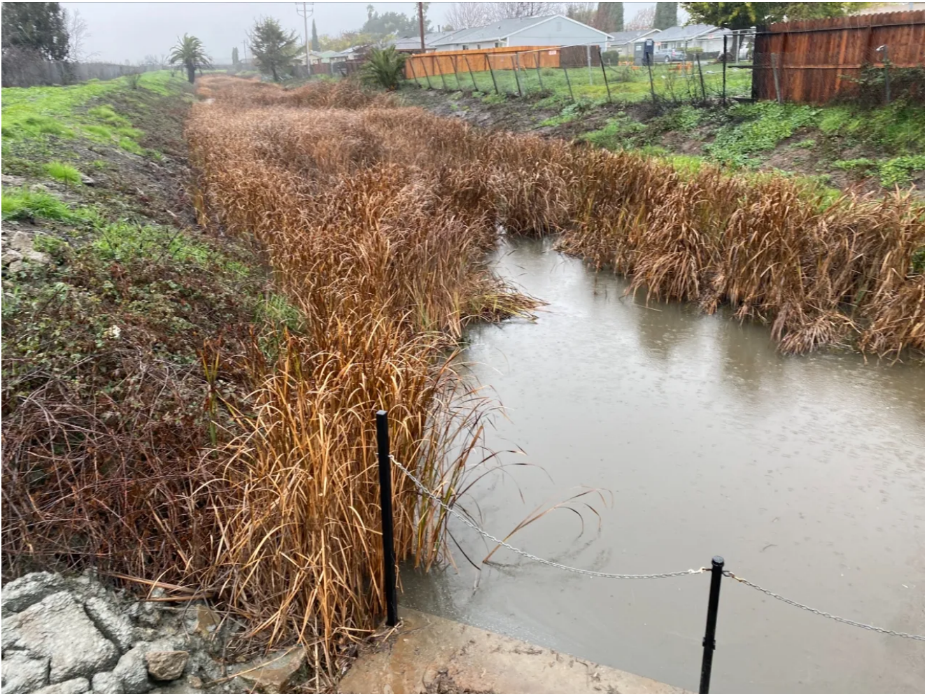
Cordelia neighborhood, burned lot, and stormwater channel. Photo: Emily Corwin.
