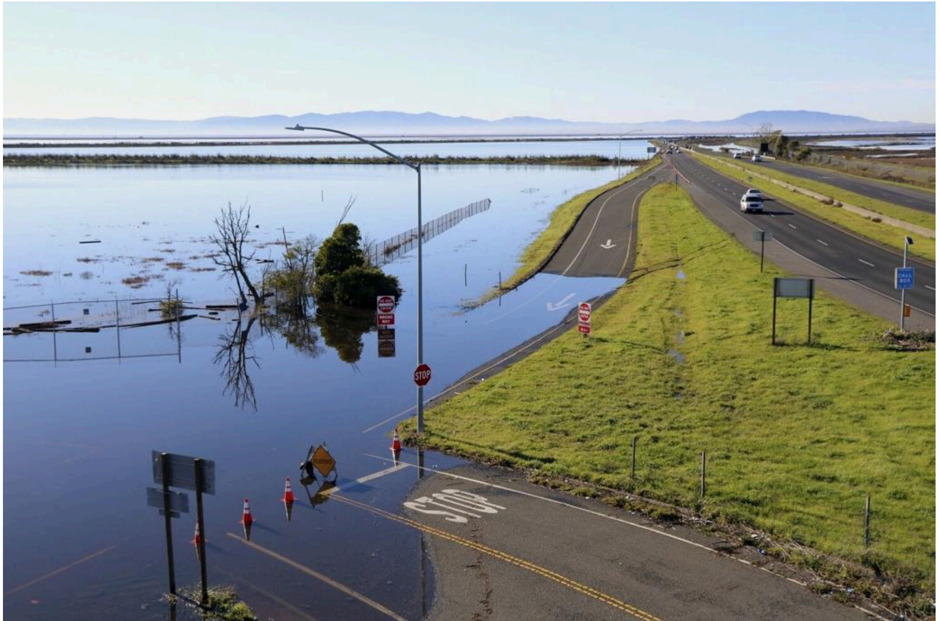
This Caltrans courtesy photos shows flooding on Highway 37, in January of 2017. (Caltrans courtesy file photo)
